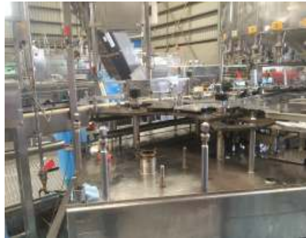
Old capping machine removed
