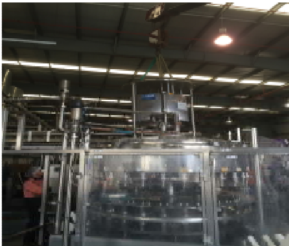
New capping machine being craned into position
